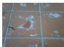
Efflorescence
